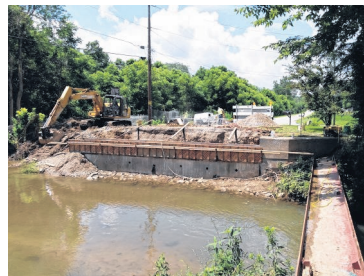
Port William Bridge Rehab
