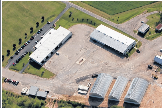
Clinton County Engineer's Office & Highway Facility
