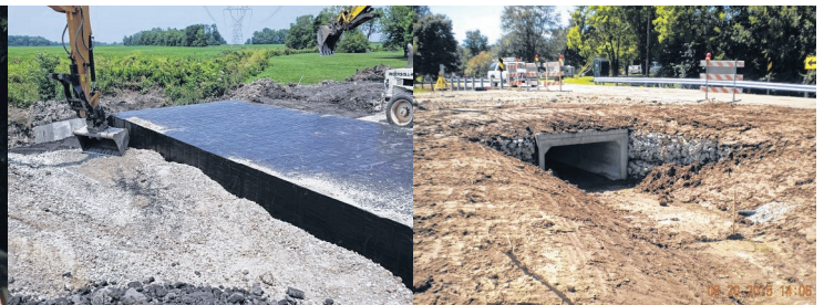
Brown Road Precast Box Culvert
